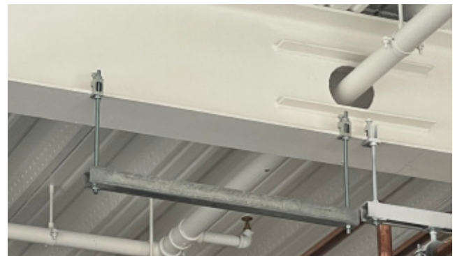
Image 17: Compliant <3000mm 2 service clips to bottom of beam, note compliant pipe penetration.
